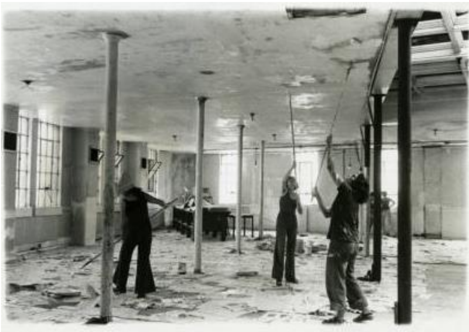
Figure 2 Women painting the ceiling on the 3rd floor of the Spring Street building, circa 1975, photo by Maria Karra, Woman's Building Ephemera, Otis College of Art and Design.
